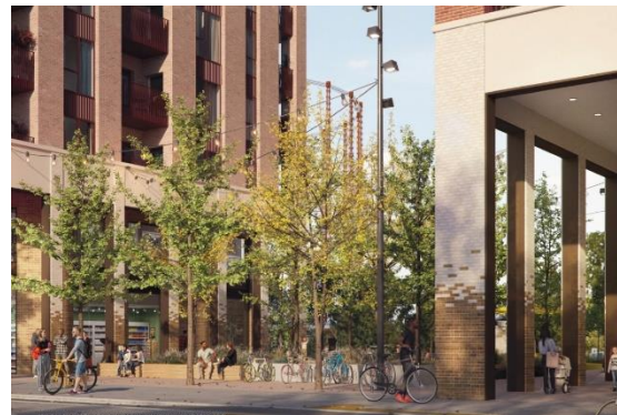
Image 74 (above): View looking through The Grove, with Gasholder 13 visible in the background.
